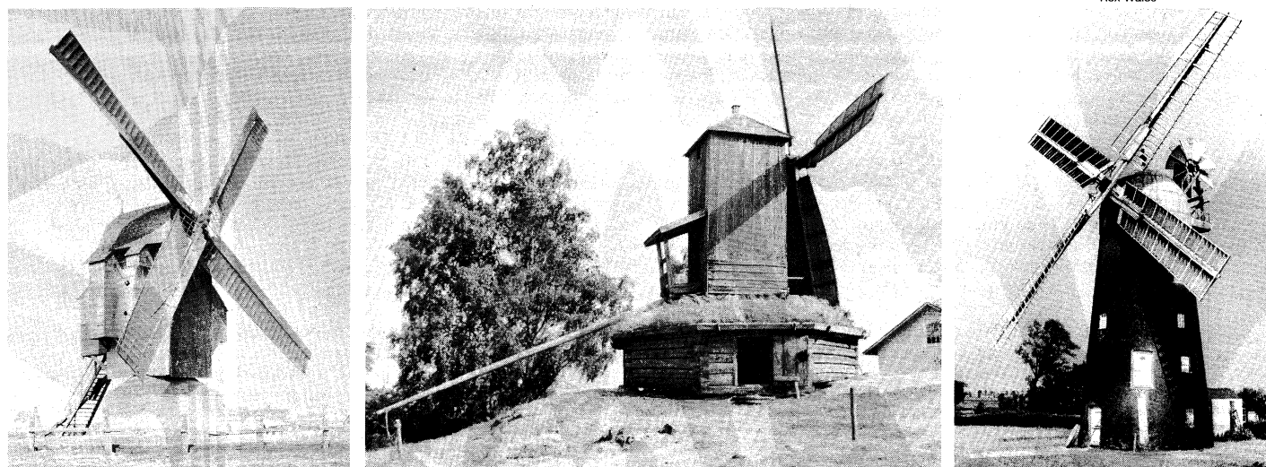
Figure 2: (Left) Post-mill with four "common sails," the cloths of which are fully set, at Marck, Pas-de-Calais, Fr. (Centre) Hollow post-mill with boarded sails, at Ylöjärvi, Häme, Fin. (Right) Tower mill with patent sails and fantail, at Pakenham, Suffolk, Eng.
